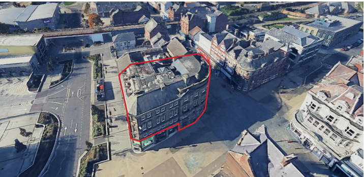
Fig 1.2.4 - Aerial view of site facing west (site boundary in red)
