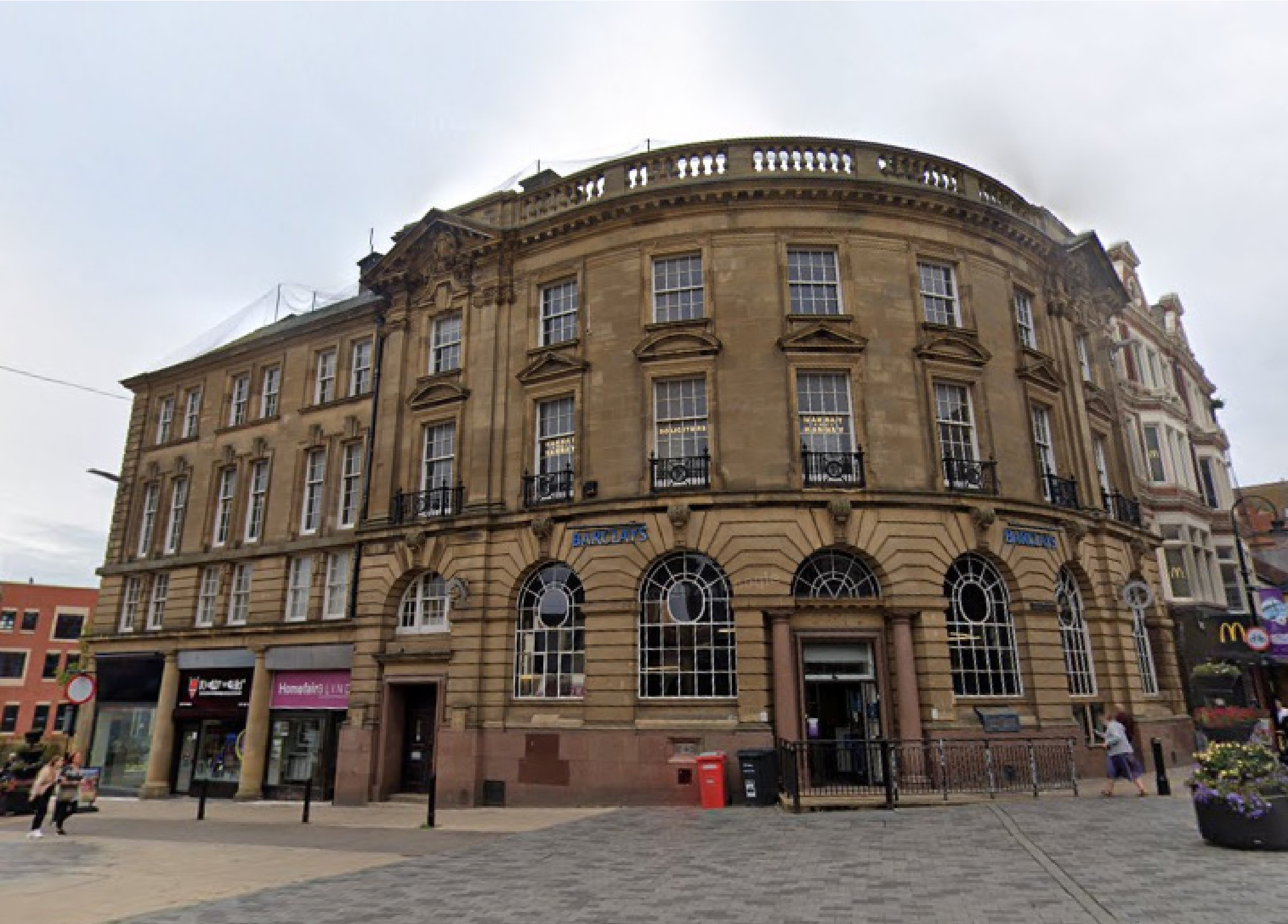
Fig 1.1.1 - Street view of front facade of building
